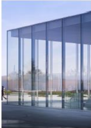
1 Ultra Clear Low Iron Transparent Glazing Faceted at the Radial Ends of the Building
