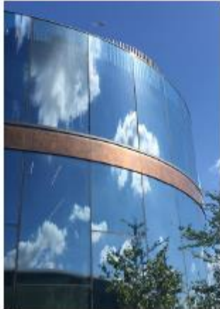
3 Double Glazed Laminated Curtain Walling with Antello Silver 70% Light Transmission Reflective Coating
