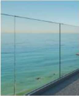
6 Structural Glazed Balustrade, Faceted to Curve
